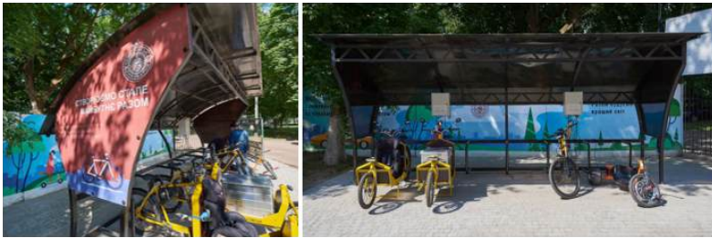
Fig. 4.5. Charging and parking station for portable electric transport
